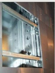
Ferrite panels are screwed onto a metallic sub-structure, made of main and secondary steel profiles. Vertical main profiles are directly fixed onto the shielded room, using the joining OMEGA profiles between two shielding panels. Then horizontal secondary profiles are screwed onto these main profiles.
